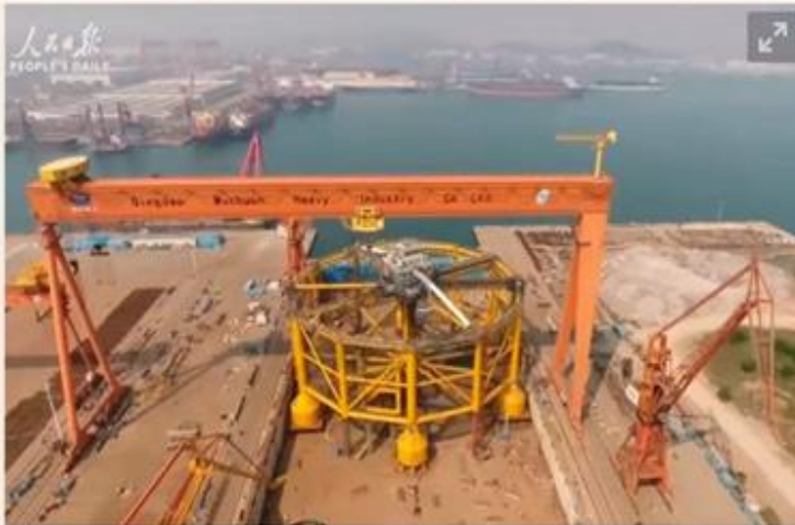
Salmor's Ocean Farm 1 under construction in Qingdao, China. Credit: People's Daily
